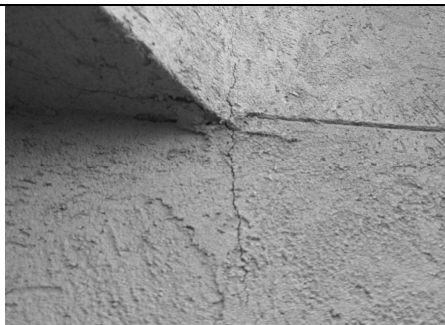
Cracking
