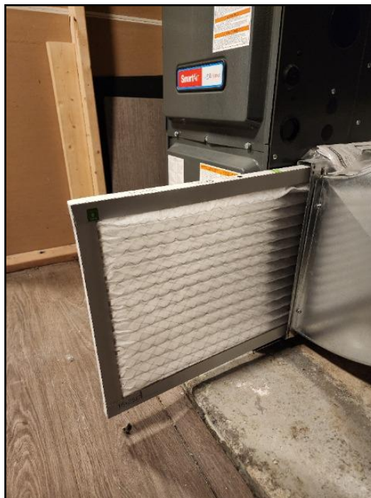
18. Replace - regular maintenance
