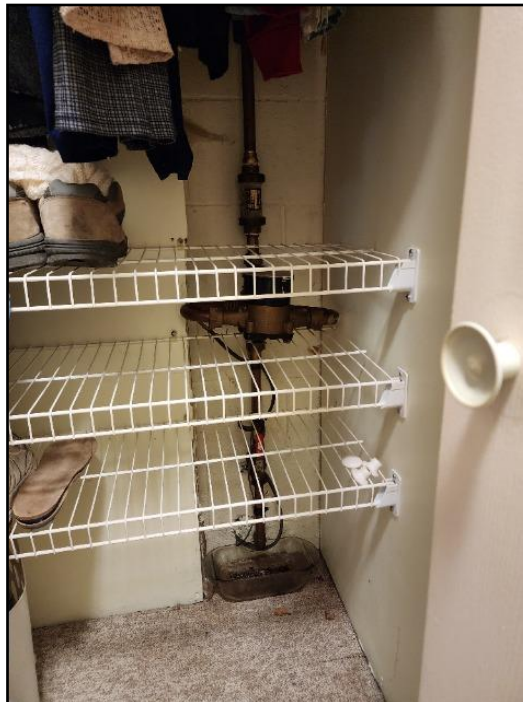
19. Main water shut off
