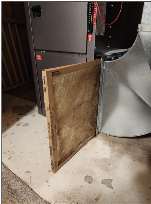
15. Replace - regular maintenance
