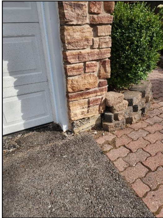
8. Spalling, crumbling or broken material
