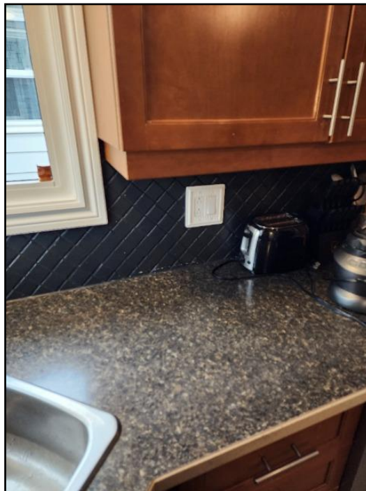
13. No GFCI/GFI (Ground Fault Circuit...
