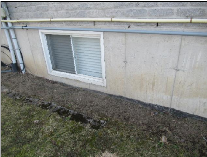
7. Typical minor cracks
