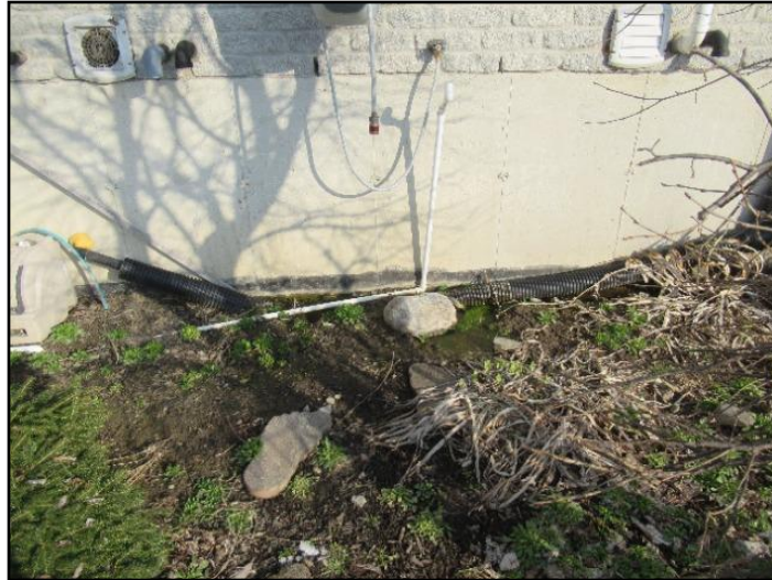
42. Discharge pipe problems
