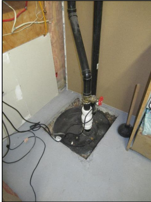
39. Solid waste pump (ejector pump)
