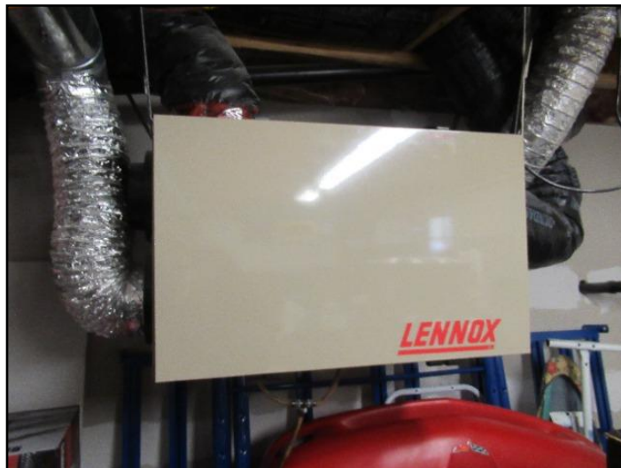
27. Heat recovery ventilator (HRV)
