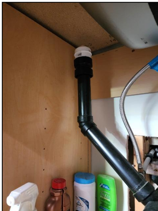
30. Automatic air vents
