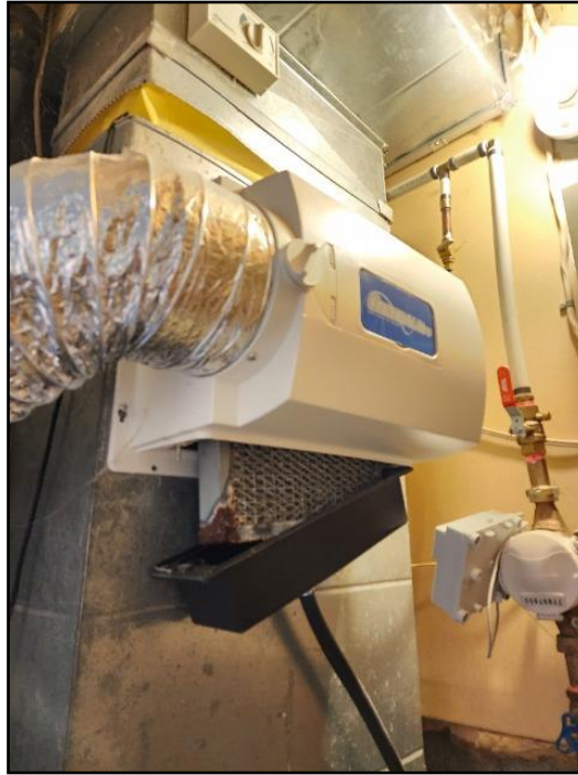
23. Clean pad/mesh - regular maintenance
