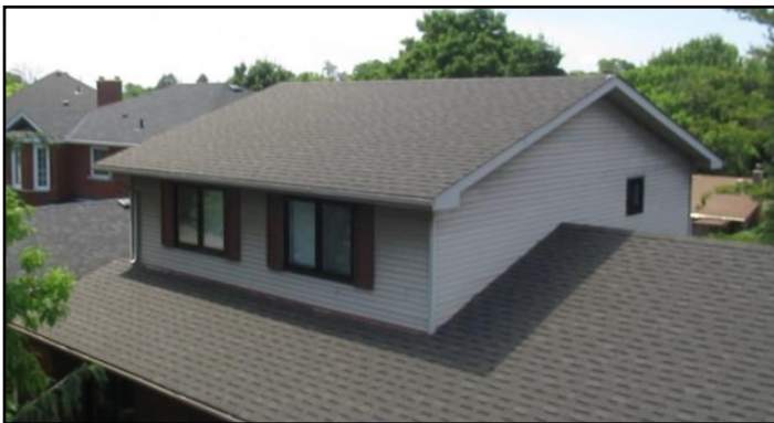
1. Asphalt shingles
