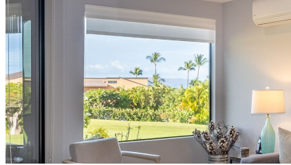
Larger living room window installed to improve view.
