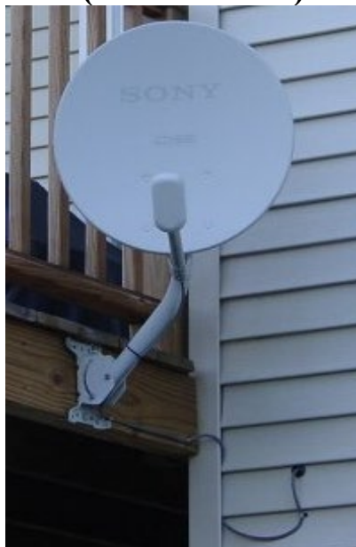
Incorrect (wires visible)
