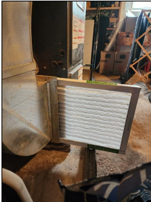
19. Replace - regular maintenance
