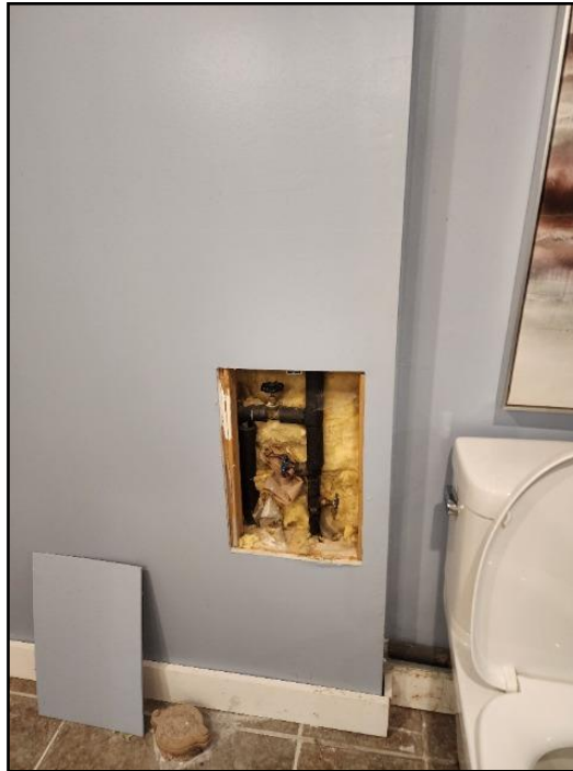
22. Main water shut off
