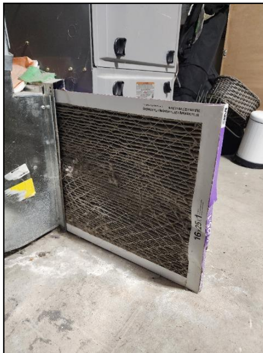
17. Replace - regular maintenance
