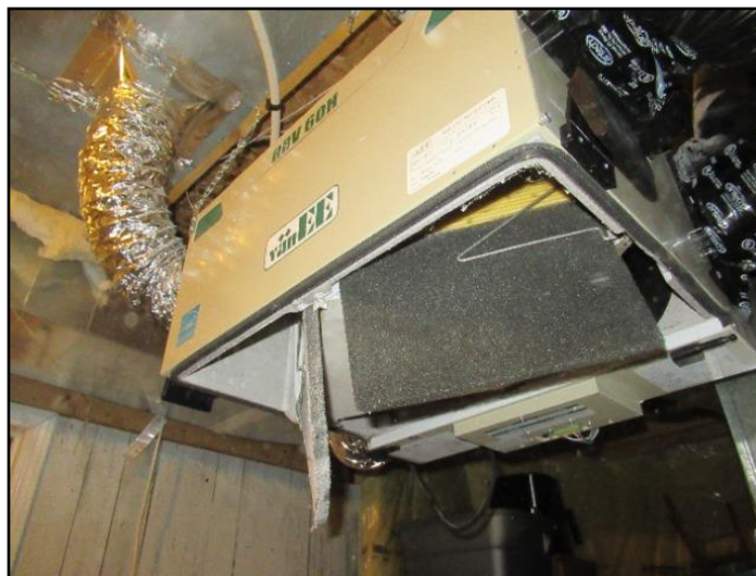
13. Clean filters - regular maintenance
