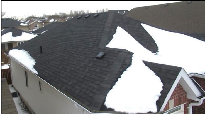
1. Asphalt shingles
