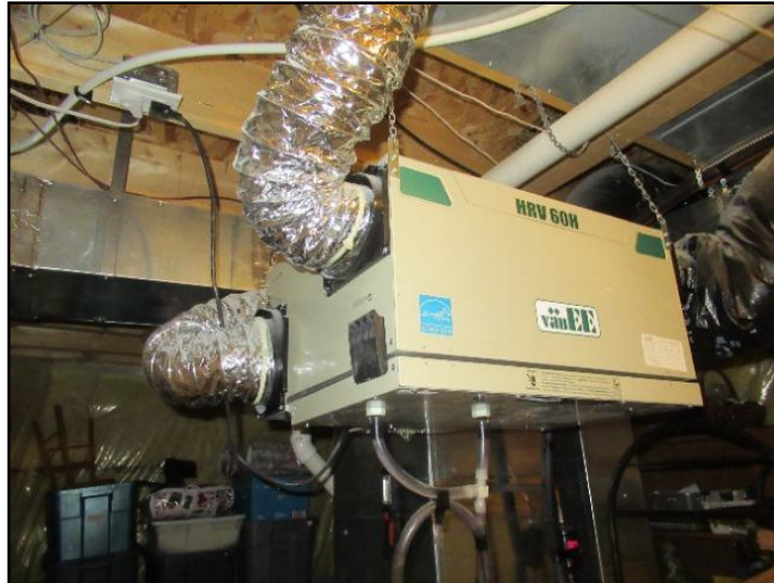
10. Heat recovery ventilator (HRV)
