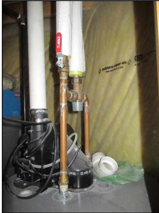
17. Tempering/mixing valve installed
