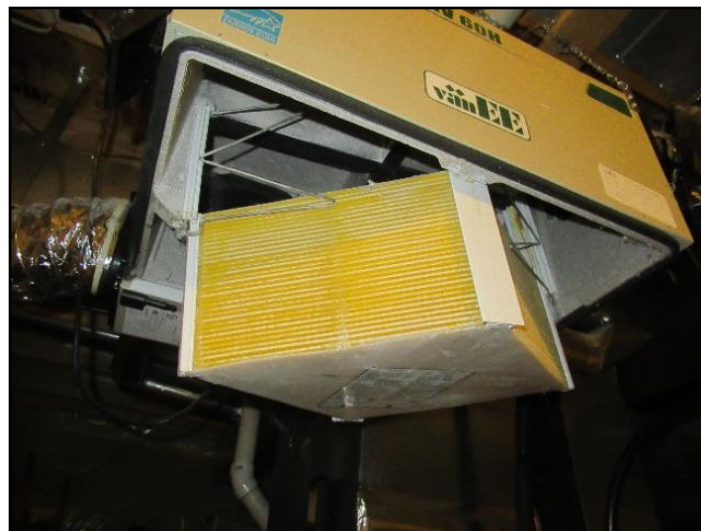
12. Clean core - regular maintenance
