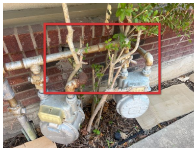
Gas piping not bonded - left exterior gas meter
