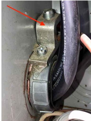
Raceway bonding clamp example
