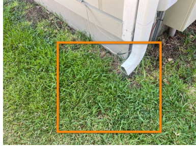
Missing splash block - rear gutter down spout
