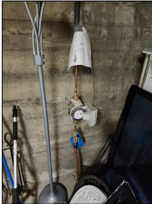
30. Main water shut off
