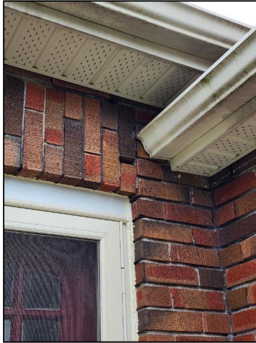
7. Masonry units moving
