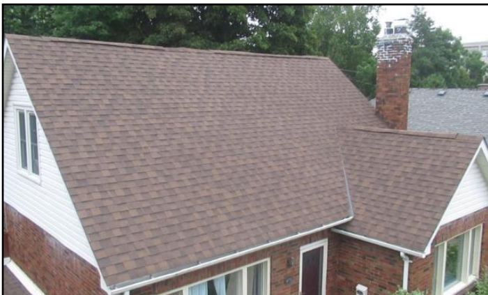
1. Asphalt shingles
