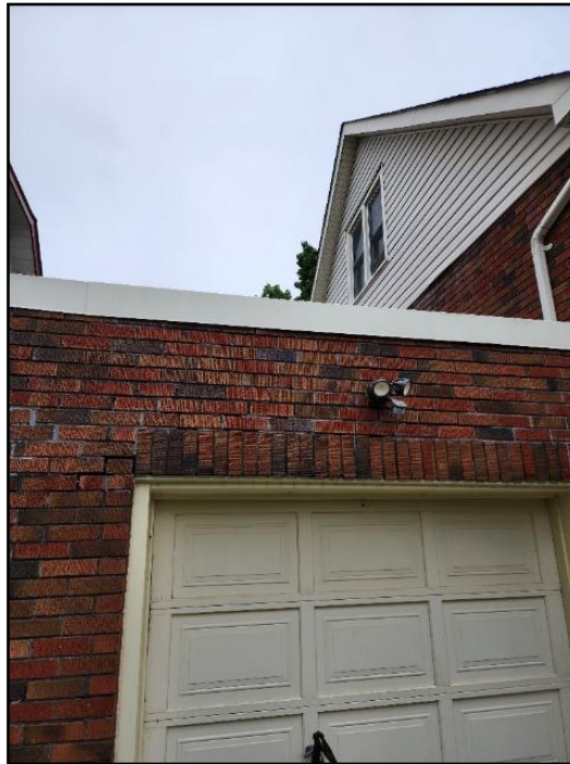
6. Mortar deteriorating
