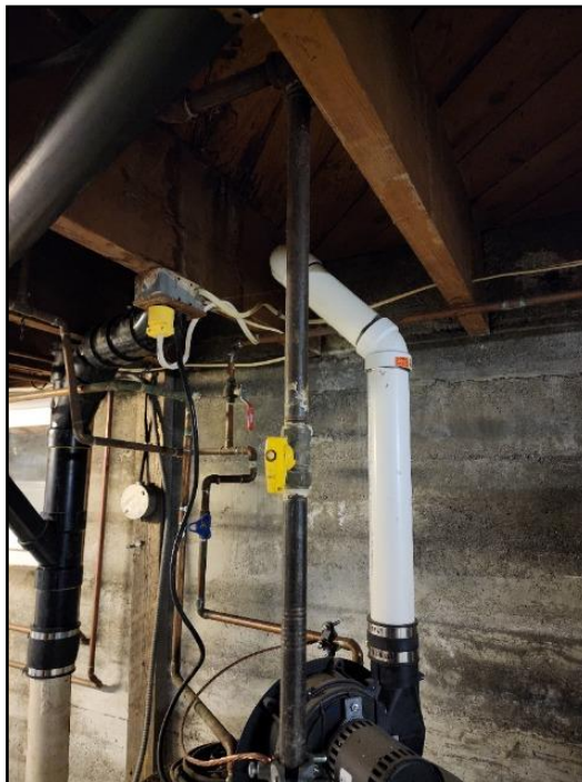
32. Main water shut off
