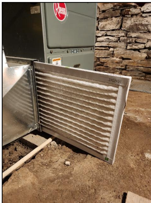
29. Replace - regular maintenance
