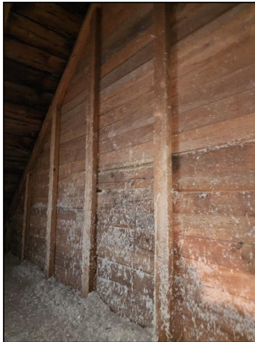
3. Extends through attic
