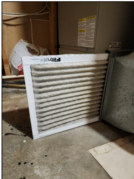
16. Replace - regular maintenance
