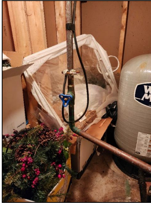
21. Main water shut off
