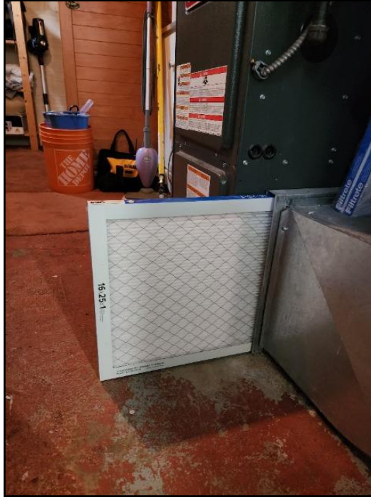
21. Replace - regular maintenance
