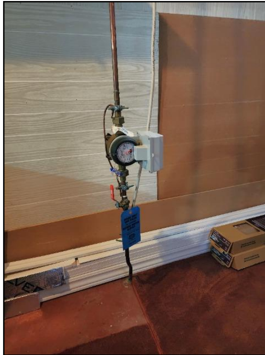
26. Main water shut off
