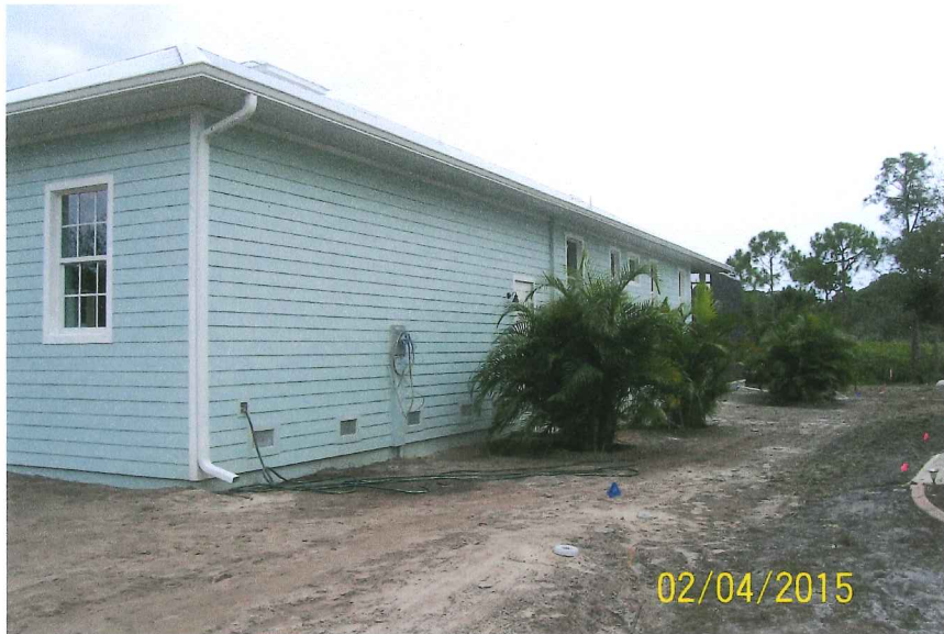
Right Side with garage vents
