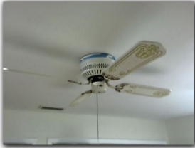
The ceiling fan is not balanced properly and wobbles when operated in middle and master bedroom.
