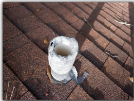
Damaged plumbing vents were observed in two or more areas. This could allow moisture to penetrate the structure.
