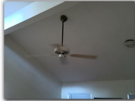
The ceiling fan is not balanced properly and wobbles when operated in middle and master bedroom.
