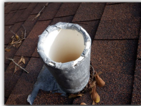
Damaged plumbing vents were observed in two or more areas. This could allow moisture to penetrate the structure.
