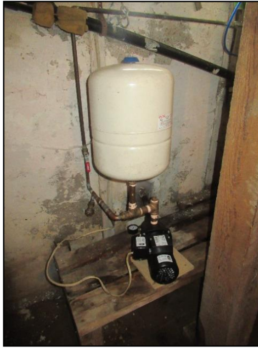
37. Well pump & pressure tank
