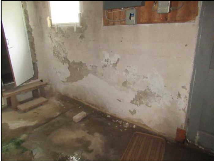
48. Crumbling/spalling masonry, concrete or...
