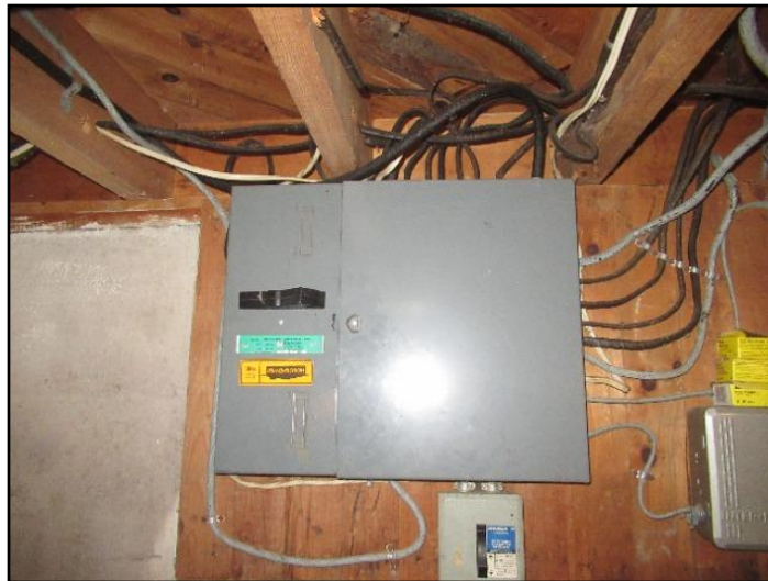
7. Main electrical disconnect
