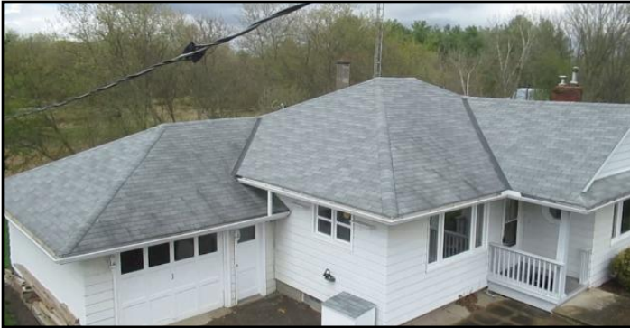
1. Asphalt shingles
