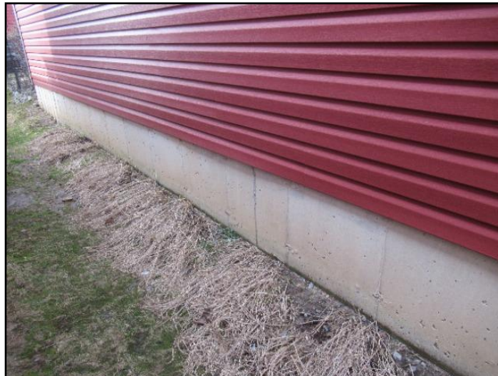
5. Typical minor cracks
