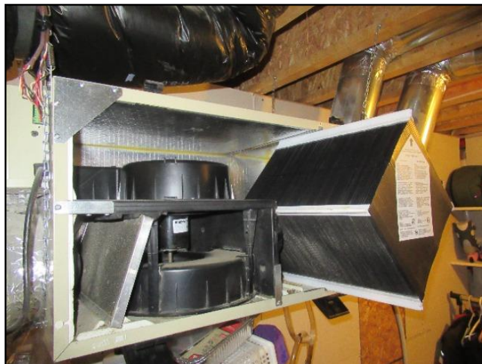
14. Clean core - regular maintenance
