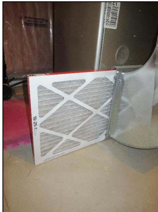
13. Installed backwards
