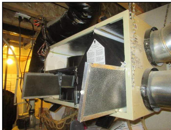
15. Clean filters - regular maintenance
