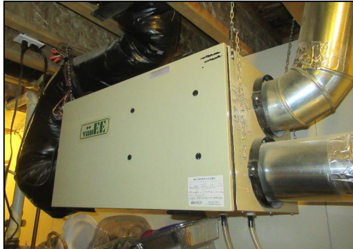
12. Heat recovery ventilator (HRV)
