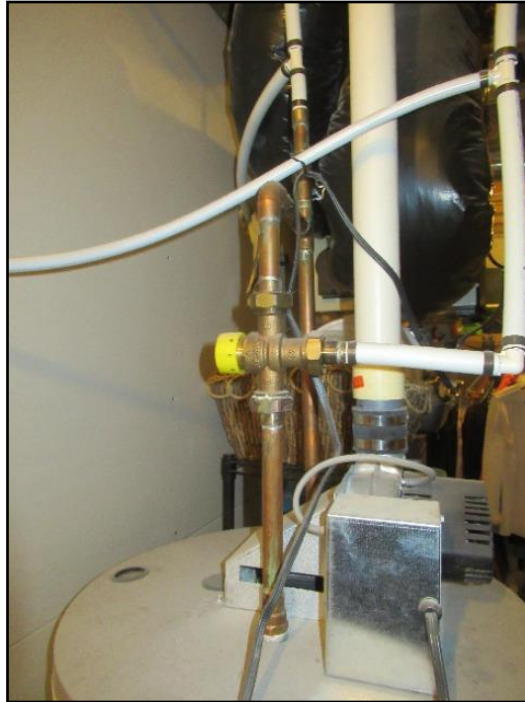
20. Tempering/mixing valve installed
