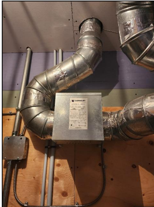
9. Electric duct heater
