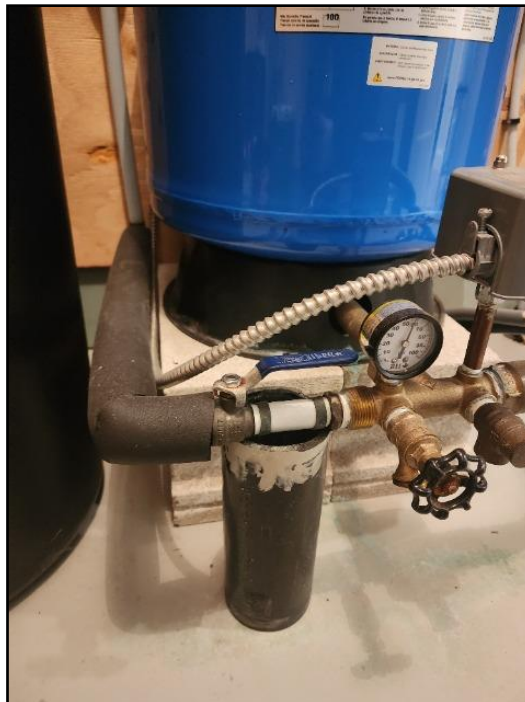
19. Main water shut off
