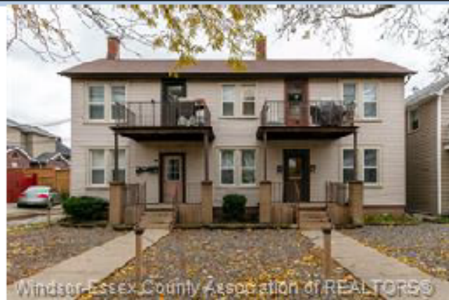
6 Plex: 2 x 2 bed & 4 x 1 bed units ; 6 x gas & 6 x hydro meters ; Unit 6 is currently Vacant $588.50 inclusive proposed
