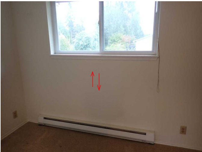
#33 Windows in S and SW bedrooms not of legal egress due to height, normal for age of house (safety).
