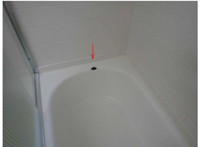
#44 Moderate chip in lower level bath enamel.
