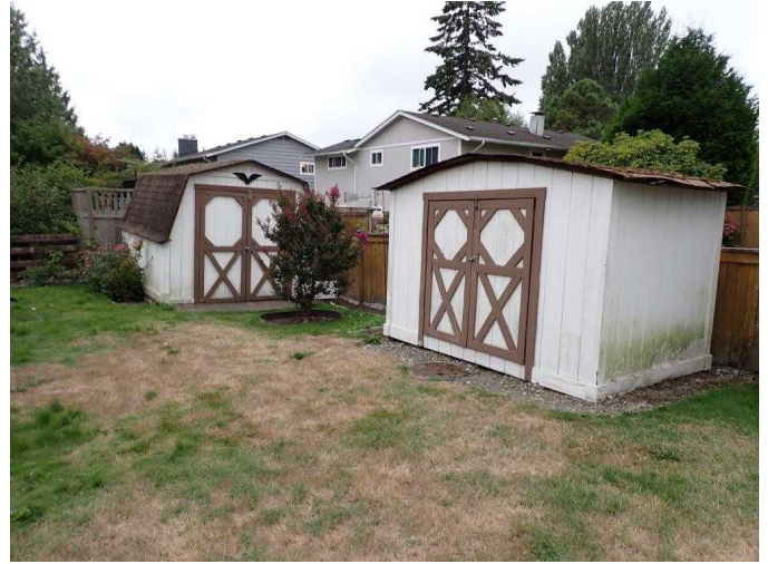
#8 Outbuildings are outside of scope of home inspection, not inspected.
