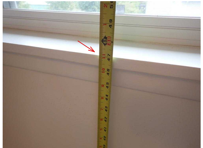
#34 Windows in S and SW bedrooms not of legal egress due to height, normal for age of house (safety).
