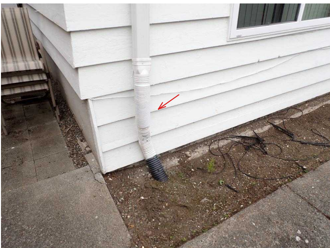
#17 Corrugated leader pipes will have a higher potential for clogging and will need to be maintained.
