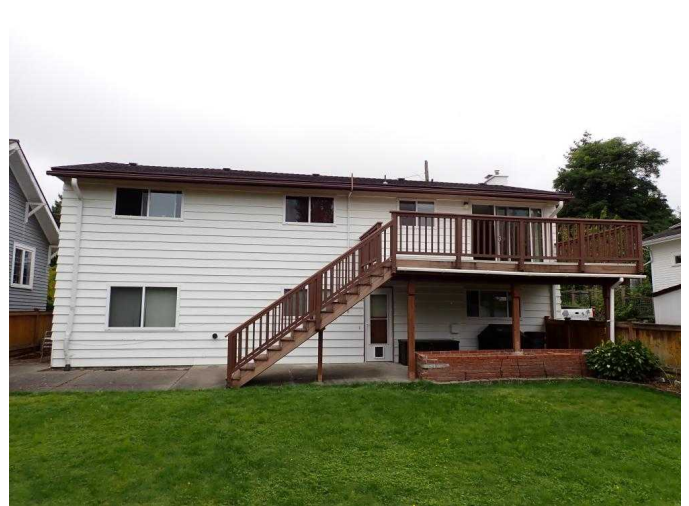
#16 S side of house.
