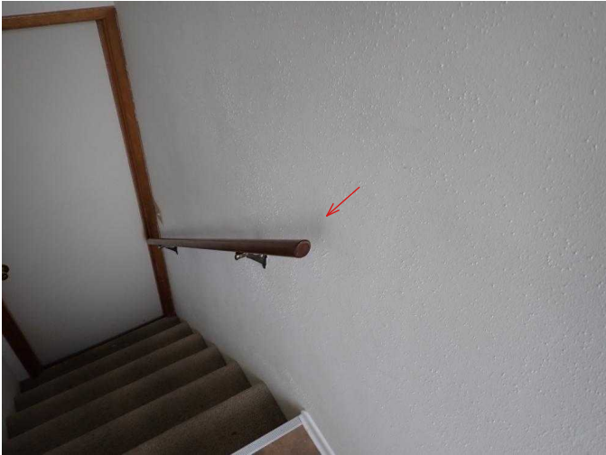
#25 No return on handrails, higher potential for articles of clothing to catch at the top end of the stairwell handrail
