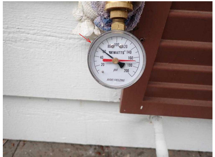
#4 Water pressure 60 psi, acceptable.
