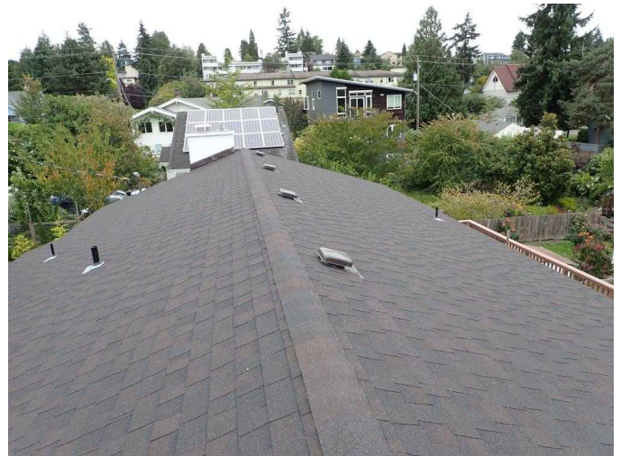
#22 Roof was fully traversed at time of inspection.
