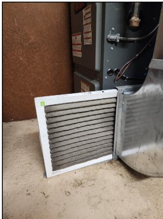
35. Replace - regular maintenance
