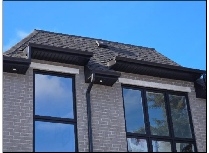
2. Asphalt shingles
