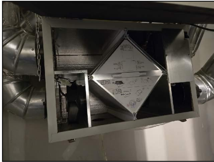
12. Heat recovery ventilator (HRV)
