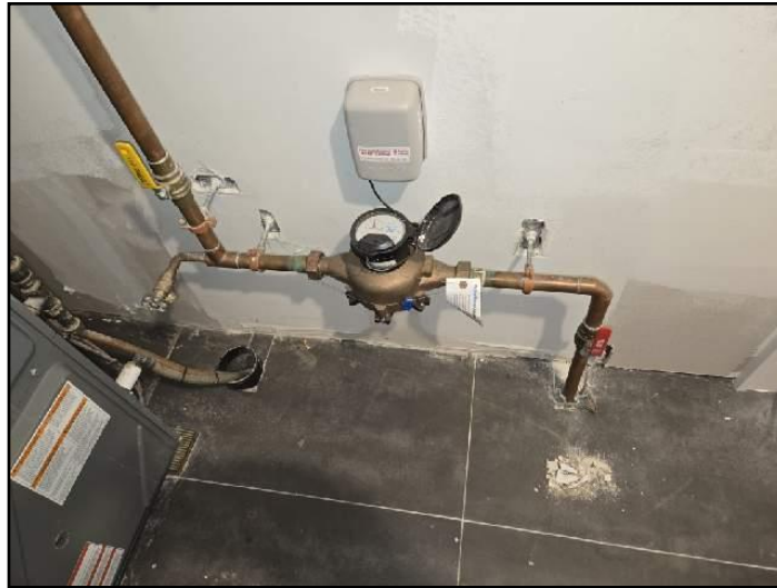
15. Water meter and shut off valve
