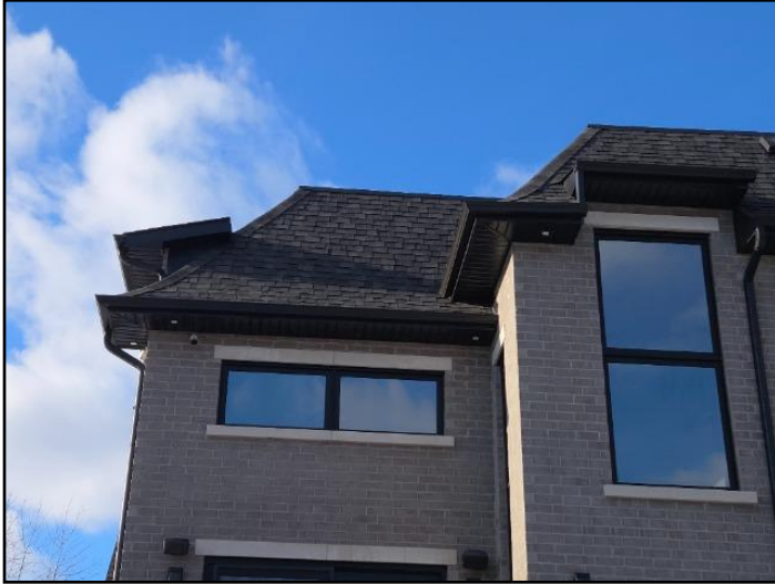
1. Asphalt shingles
