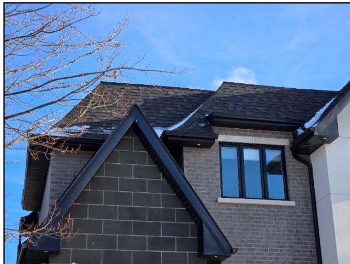
3. Asphalt shingles
