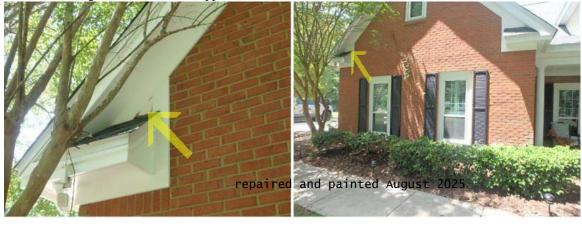
8. Rot and deterioration noted at the front garage window trims here.
