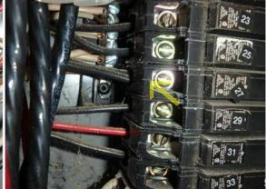
37. Missing wire connector / clamp noted at the electrical sub-panel where wiring has been added.
