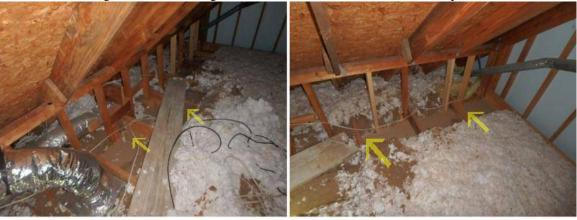
26. Moisture staining / rot noted at the roof decking around the main house chimney. Damaged areas tested dry at time of inspection. Recommend monitoring.
