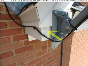
14. Deterioration / chipping and flaking noted at the rear upper window trims.
