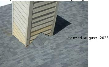
22. The fresh air return vent termination piece is missing at the right side chimney above the roof level.
