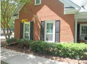
6. Separation and evidence of settlement noted at the right side exterior shed addition. Separation noted at the brick mortar at the transition to the house. Brick coursing does not appear level at the front facing wall.
