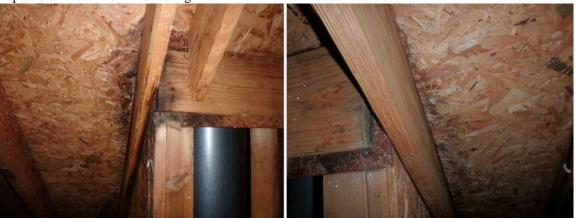
27. Moisture staining / rot noted at the roof decking around the addition area chimney. Damaged areas tested dry at time of inspection. Recommend monitoring.
