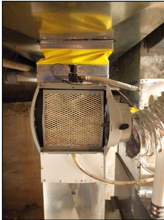
27. Clean pad/mesh - regular maintenance
