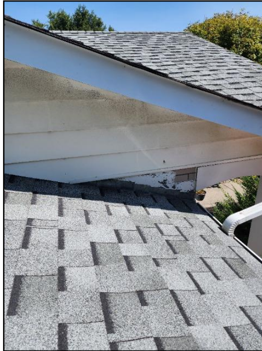
4. No step or counter flashings
