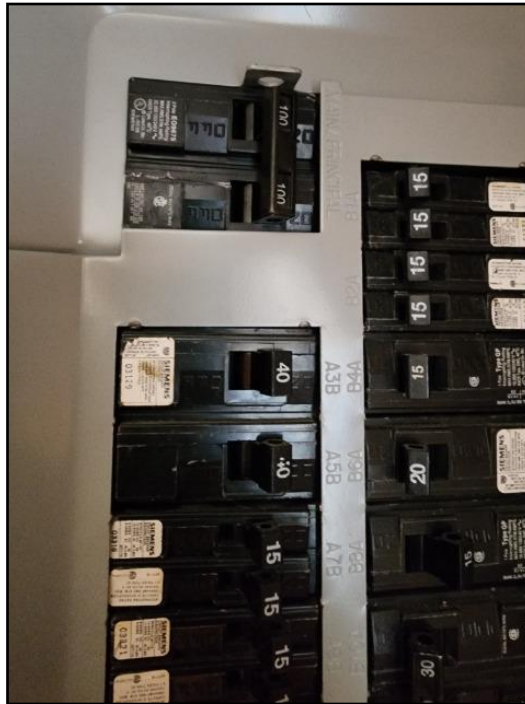
16. Breaker bridge missing
