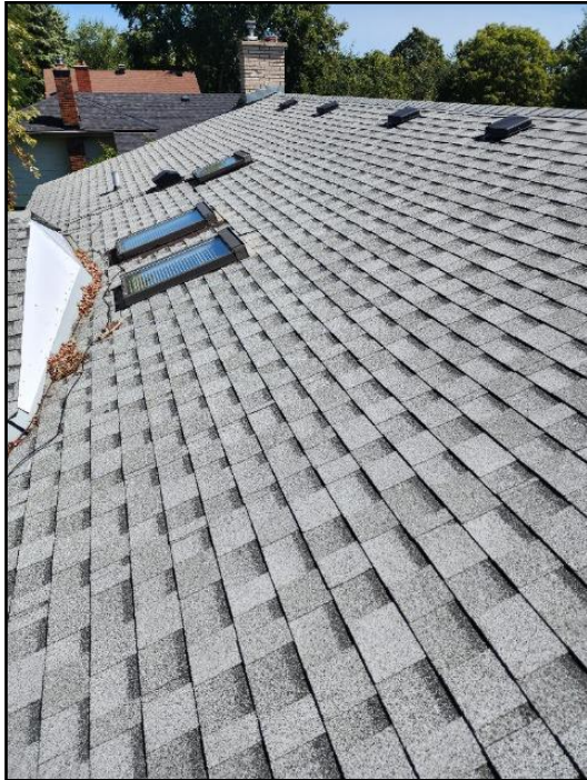
1. Asphalt shingles
