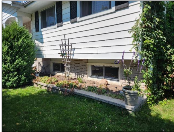
12. Masonry or wood too close to grade
