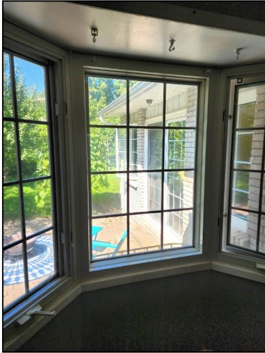
43. Lost seal on double glazing
