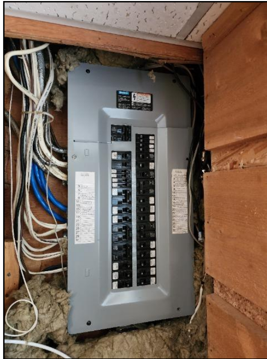
13. Main electrical disconnect
