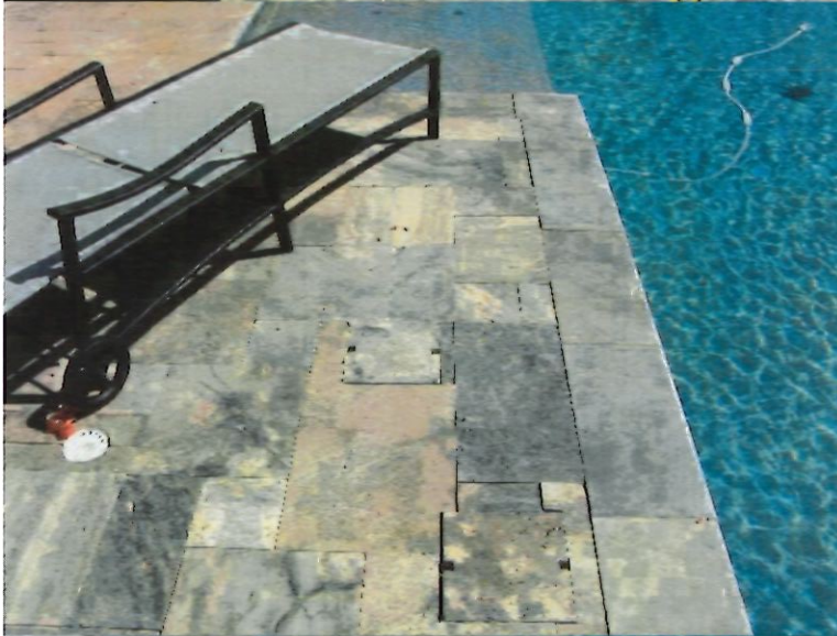
44. Southwest perimeter of pool where water line tiles have been replaced.
