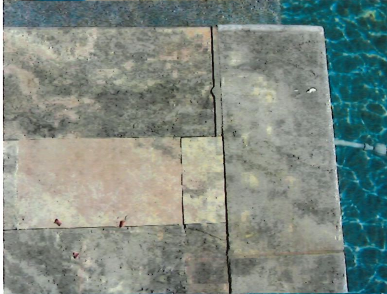
47. Southwest perimeter of pool where water line tiles have been replaced.
