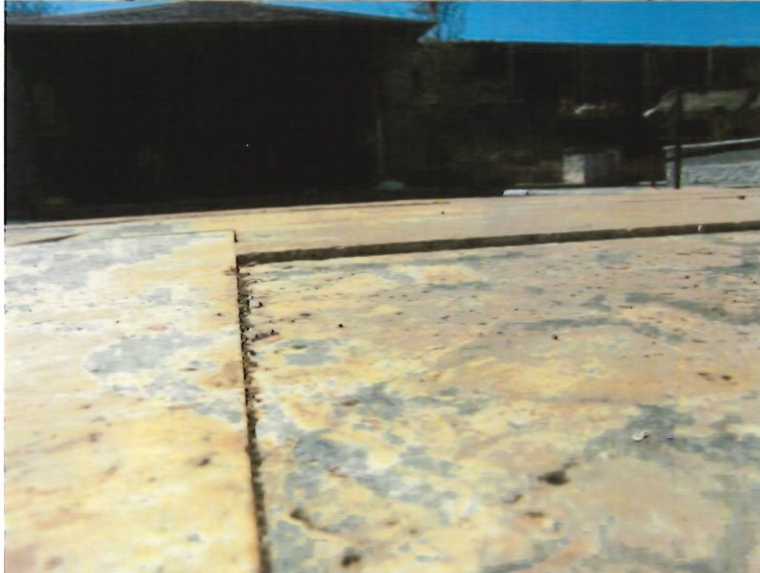
33. Diselevation of paver along west side of tanning ledge.
