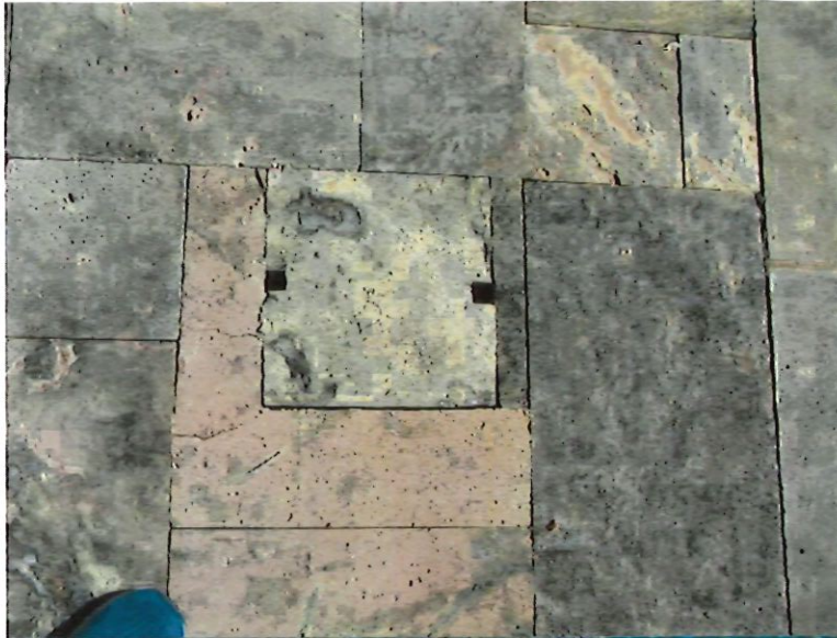
46. Southwest perimeter of pool where water line tiles have been replaced.
