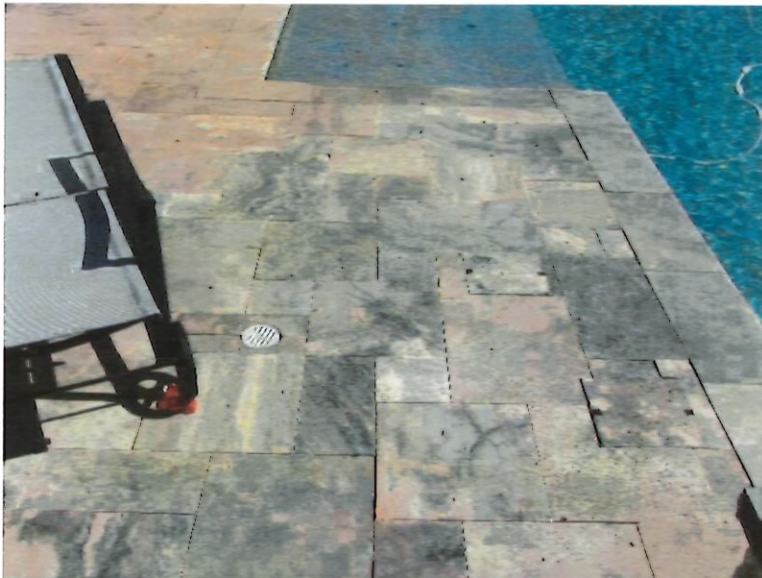
49. Southwest perimeter of pool where water line tiles have been replaced.
