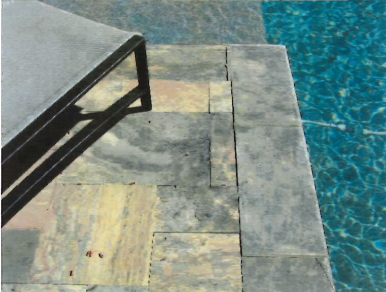
45. Southwest perimeter of pool where water line tiles have been replaced.
