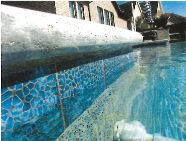
37. Opposite side of corner of prior photograph.
