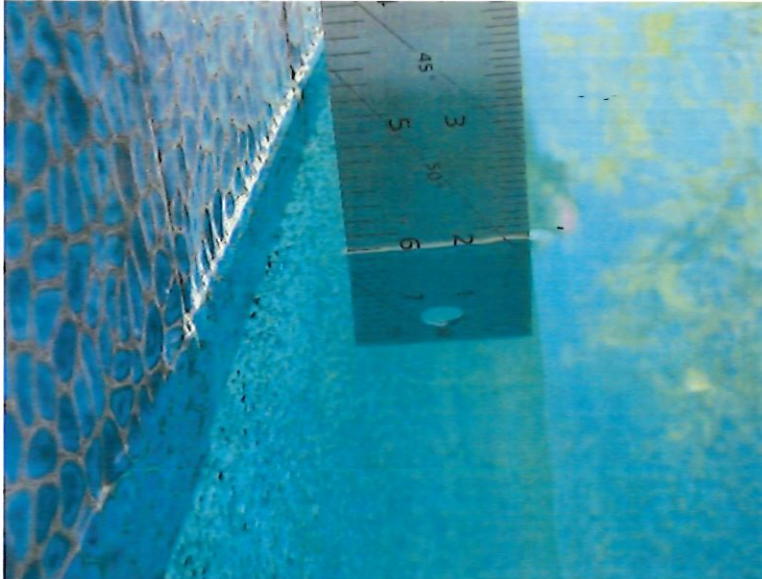
10. Water level at quarter point from south perimeter, east side, measures 6-1/8" below top of coping.
