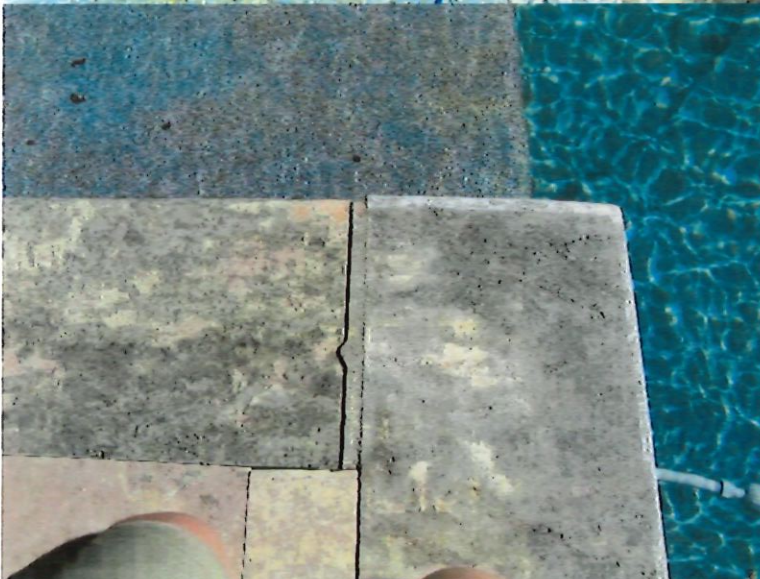
36. Top view of prior photograph.
