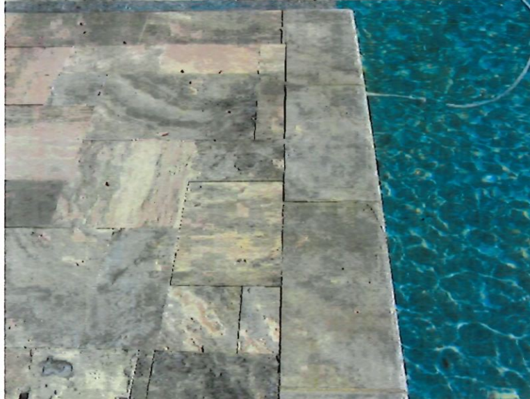
48. Southwest perimeter of pool where water line tiles have been replaced.
