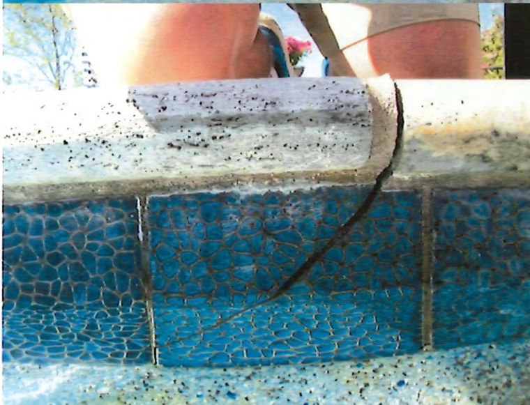
35. Close-up view of prior photograph.
