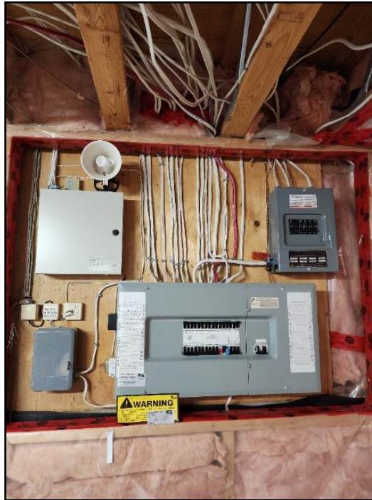
3. Main electrical disconnect
