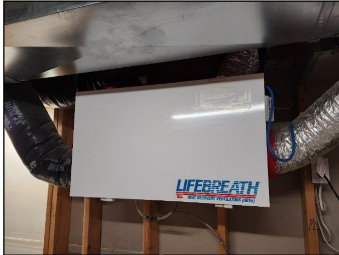
18. Heat recovery ventilator (HRV)
