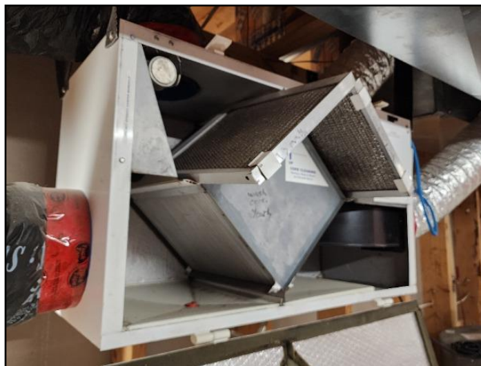
21. Clean filters - regular maintenance
