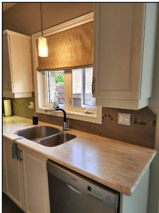
8. No GFCI/GFI (Ground Fault Circuit...
