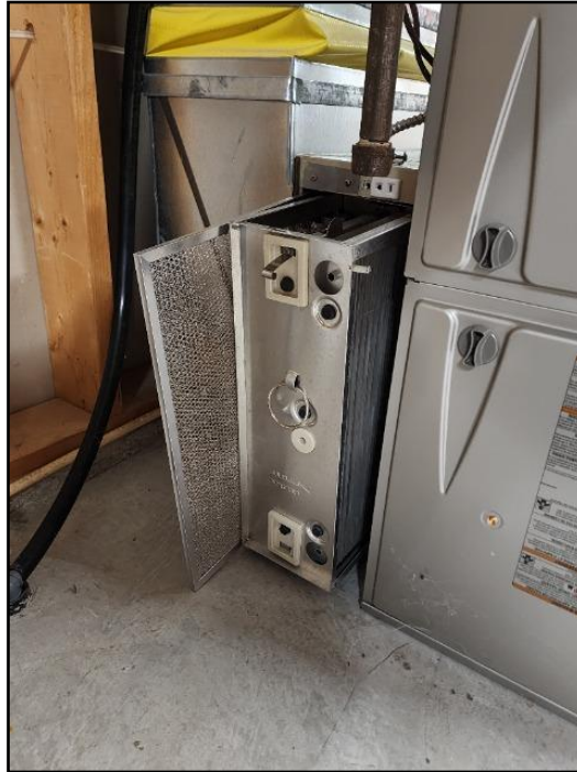
19. Clean cells/filters - regular maintenance
