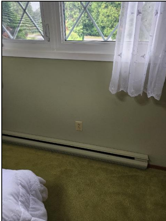
22. Electrical receptacle above heater
