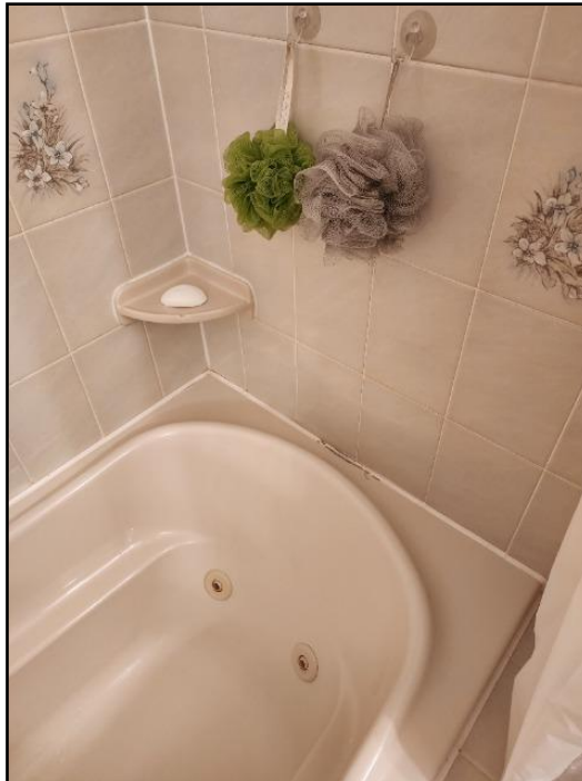
34. Caulking loose, missing or deteriorated
