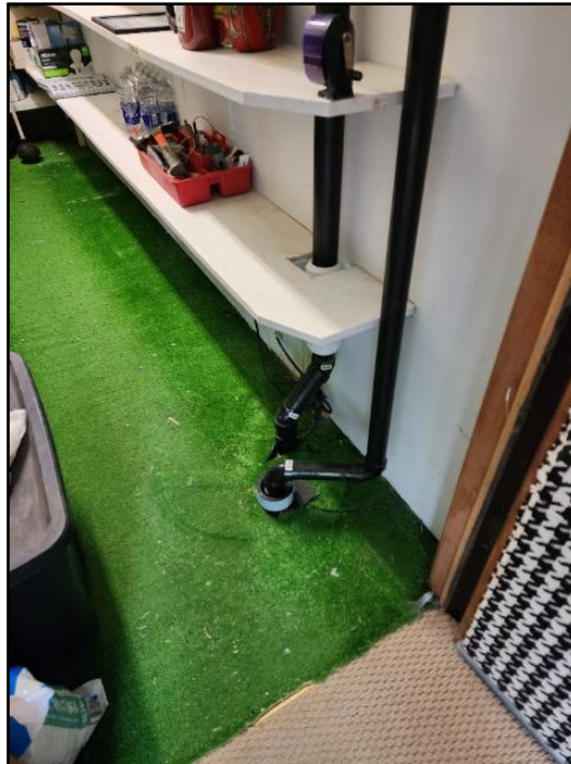
30. Solid waste pump (ejector pump)
