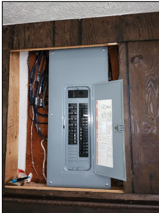
6. Main electrical disconnect
