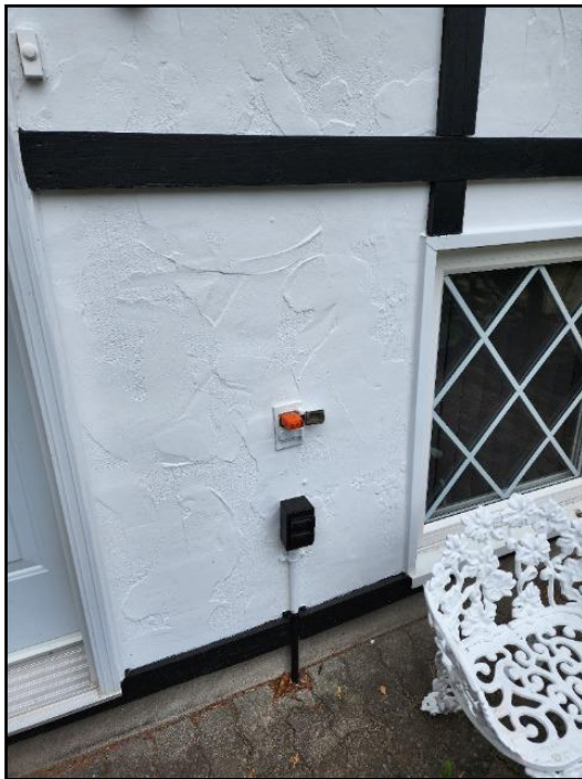
11. No GFCI/GFI (Ground Fault Circuit...
