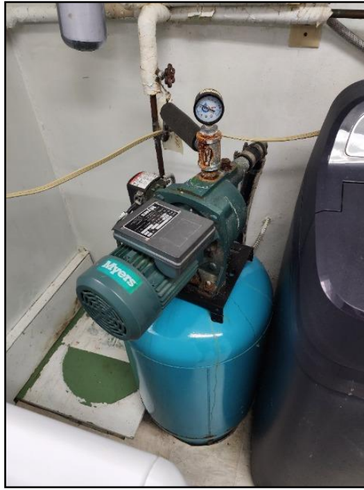
25. Well pump & pressure tank
