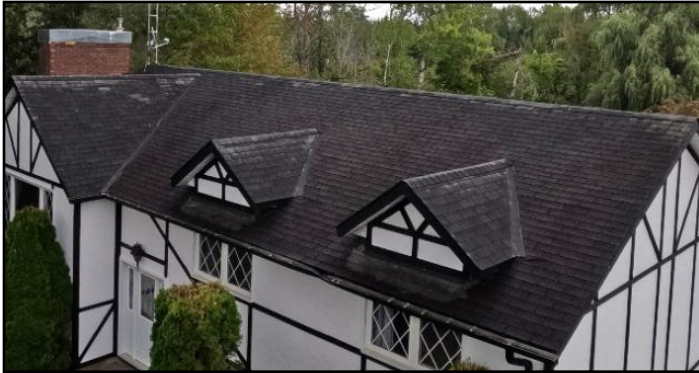
1. Asphalt shingles
