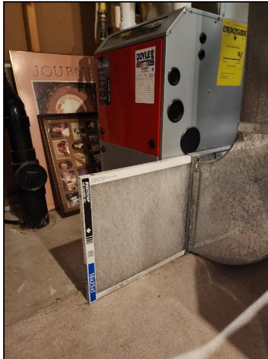
15. Replace - regular maintenance
