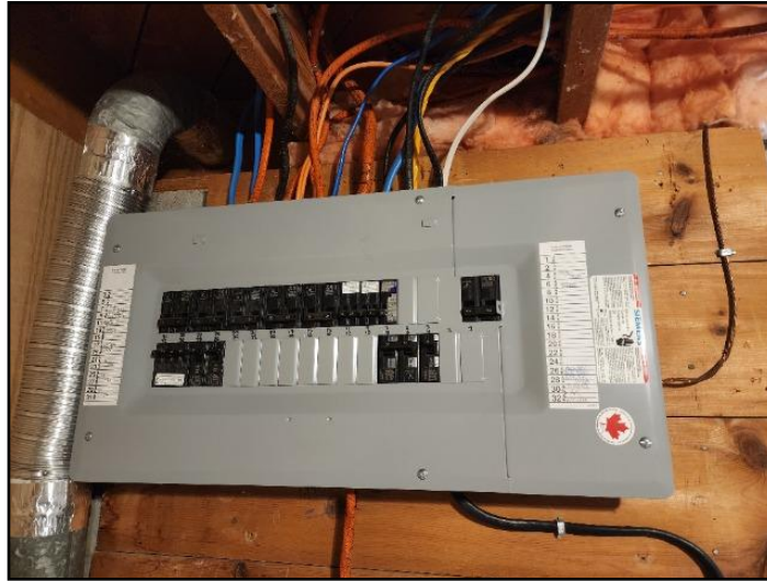
5. Main electrical disconnect
