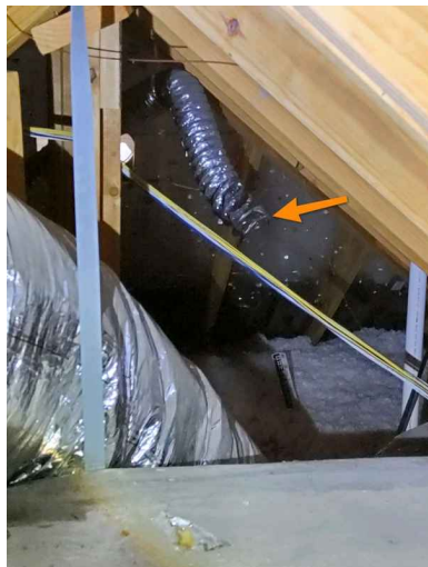
East Side Of The Upper Level Attic
