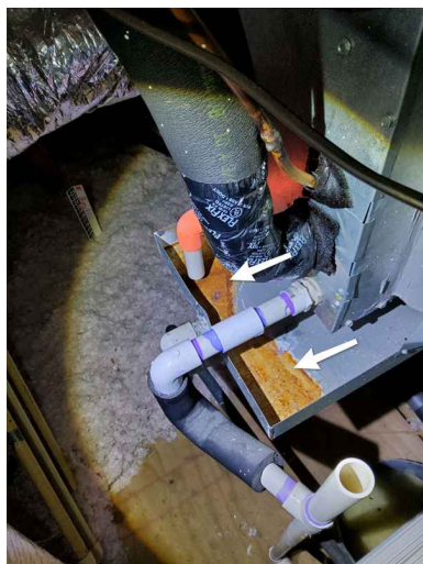
West Unit In The Attic
