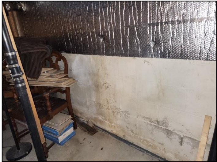
32. Efflorescence
