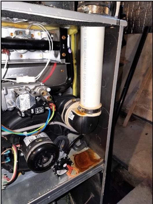
22. Condensate problems/leak
