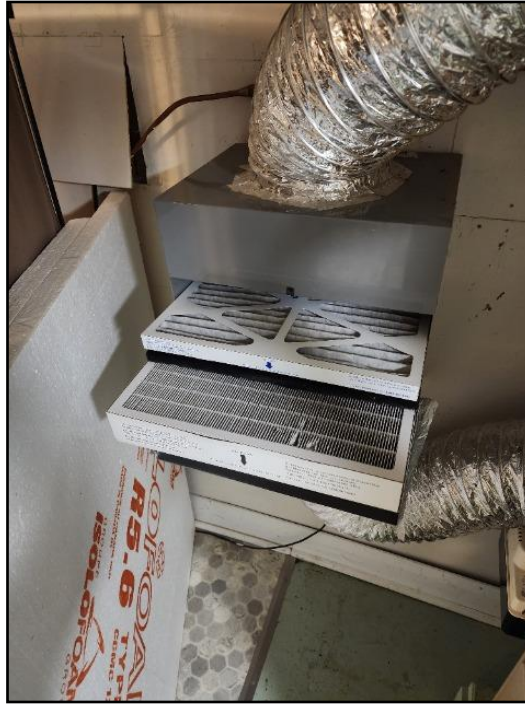
30. Replace - regular maintenance
