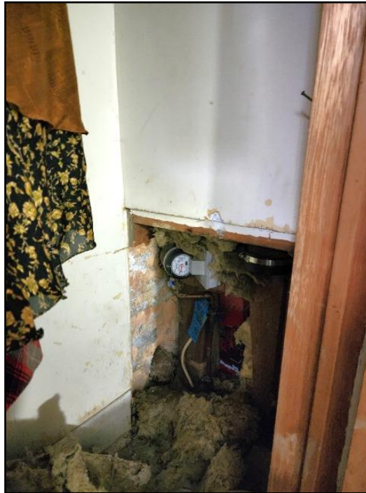
35. Main water shut off
