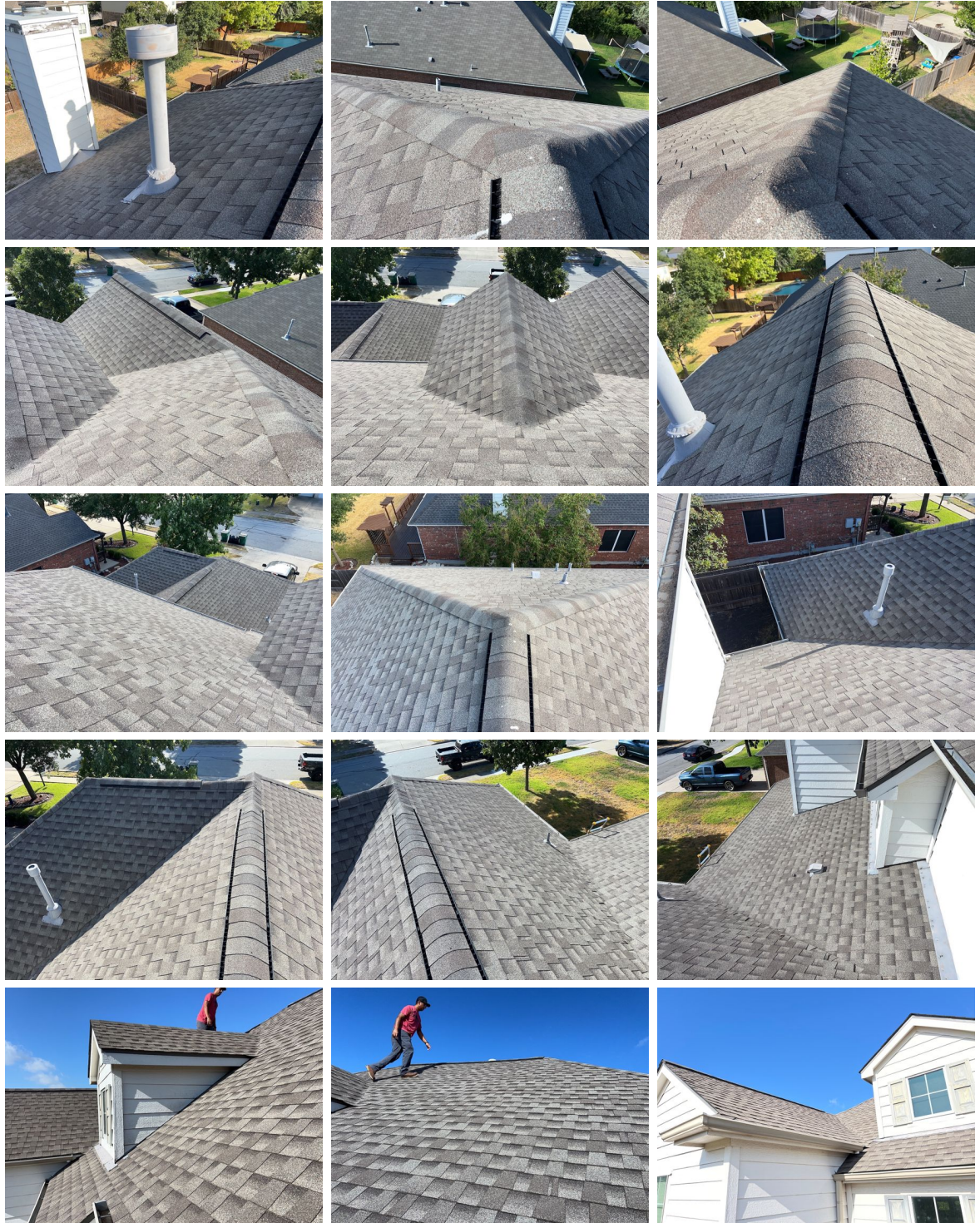
Photos - Average roof condition photos (See below photos):
