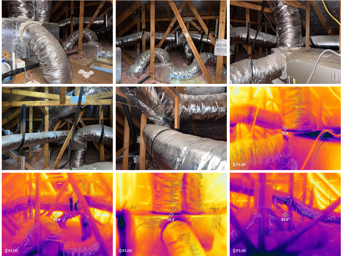
Photos - Ducts and Thermal Images Taken During Operation (See below photos):
