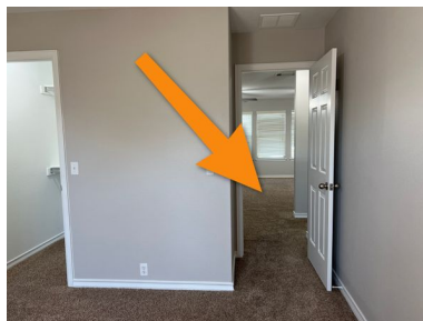
2nd Floor Front Left Bedroom
