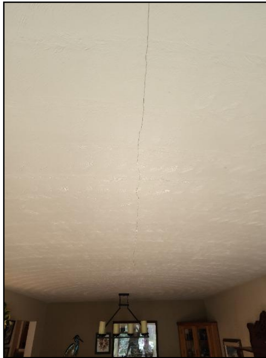
35. Minor cracking
