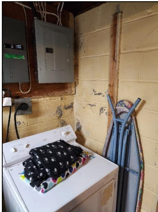
37. Efflorescence
