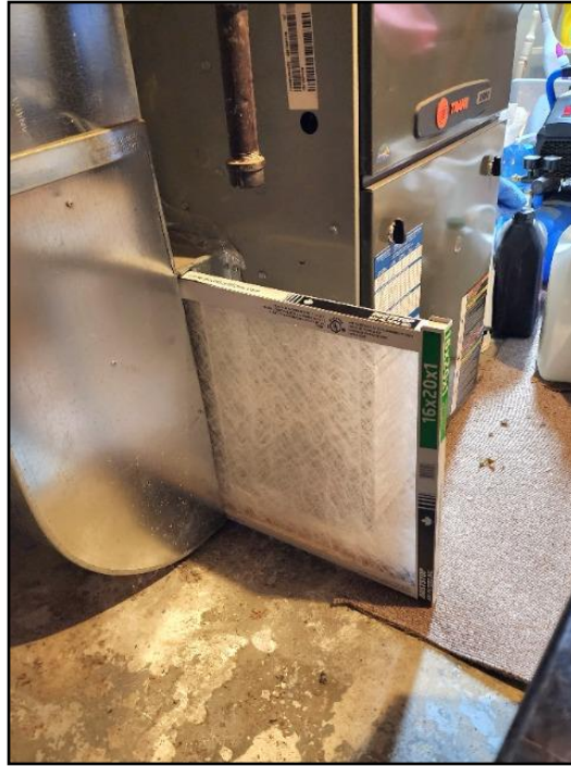
25. Replace - regular maintenance
