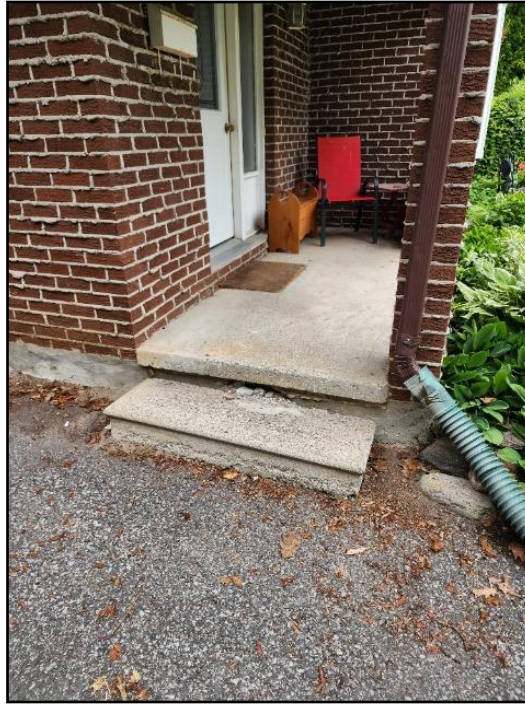
5. Concrete spalling
