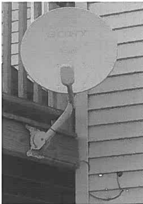
Incorrect (wires visible)
