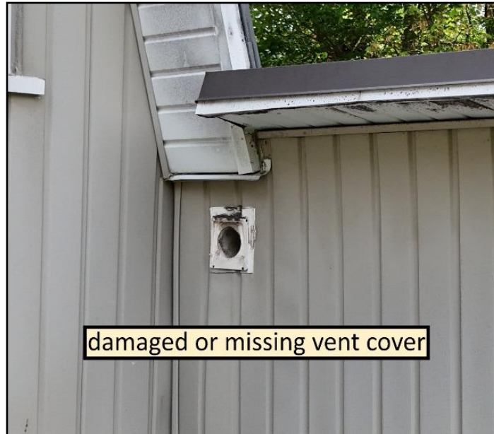
38. Vent cover missing or damaged.
