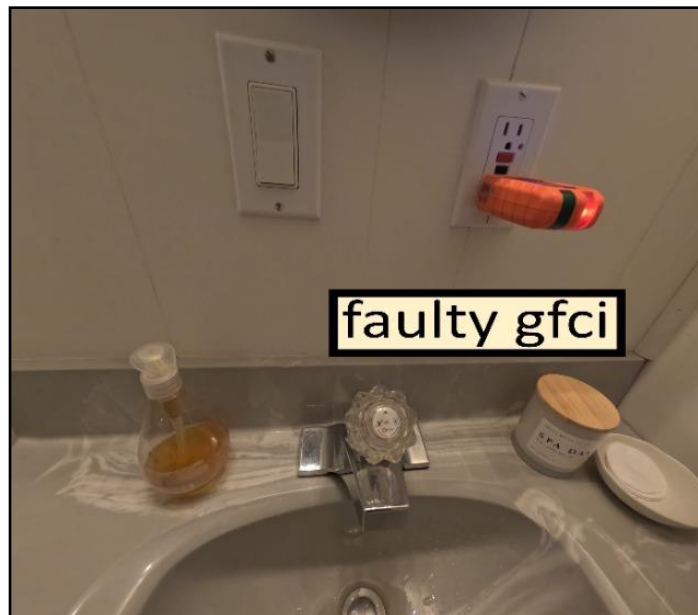
50. Test faulty on GFCI/GFI (Ground Fault...
