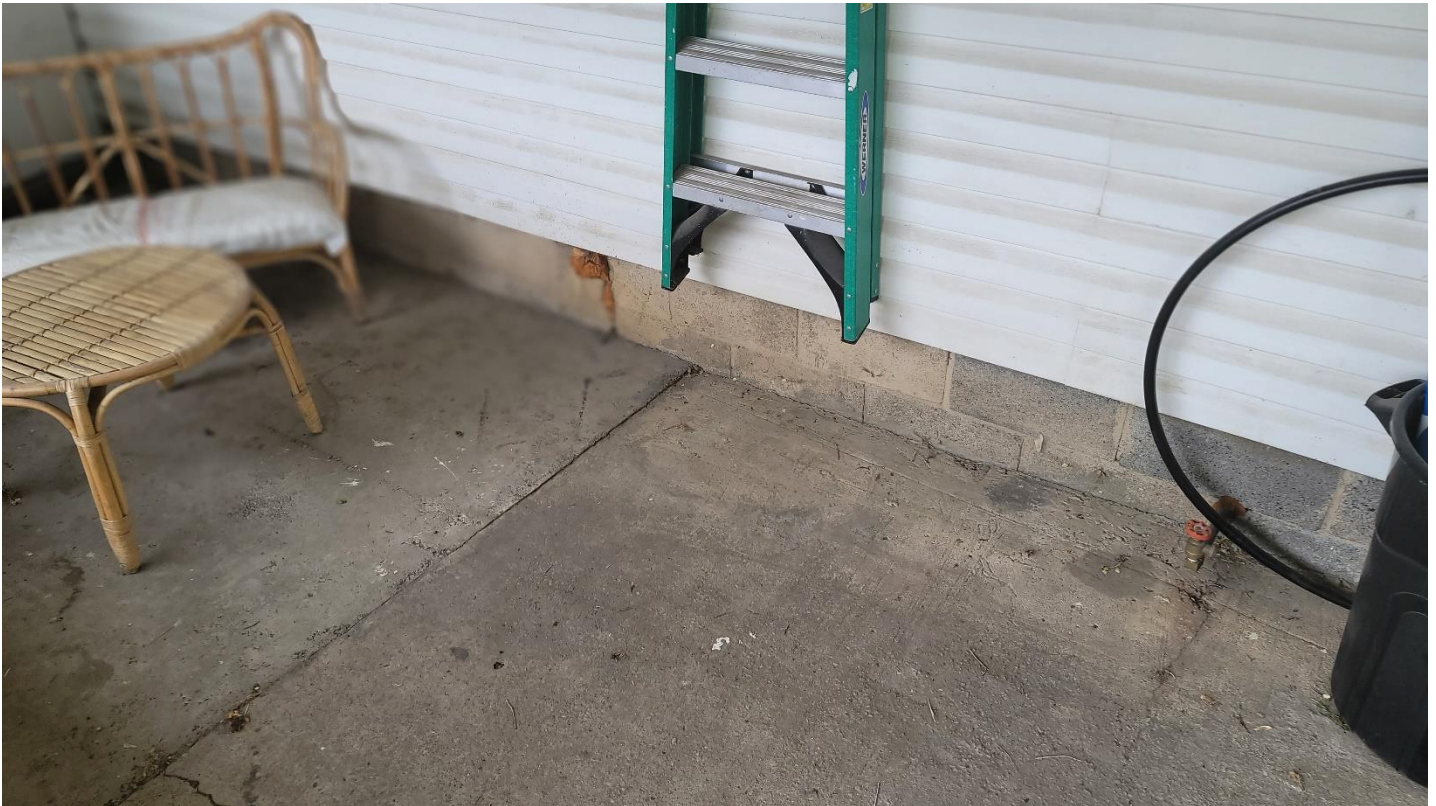
The addition on the back side uses a block foundation
