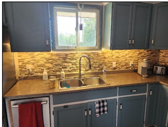
13. No GFCI/GFI (Ground Fault Circuit...
