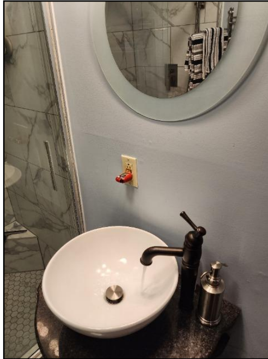
14. Test faulty on GFCI/GFI (Ground Fault...
