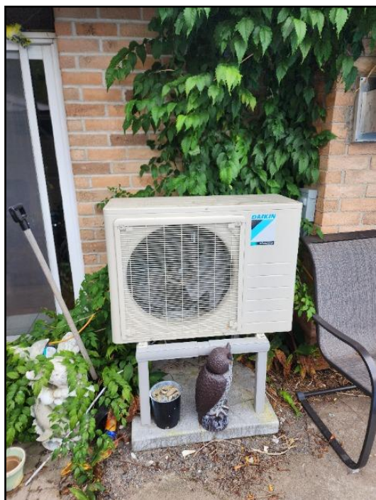
20. Ductless (Mini split) system
