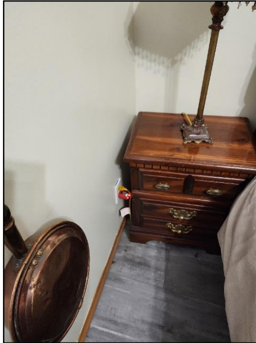
11. Reversed polarity
