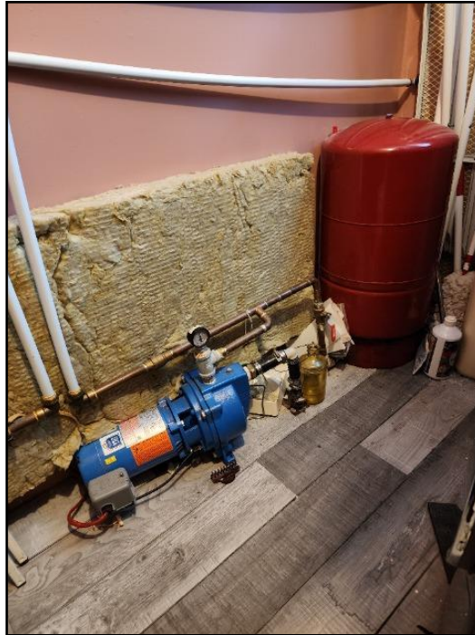
23. Well pump & pressure tank
