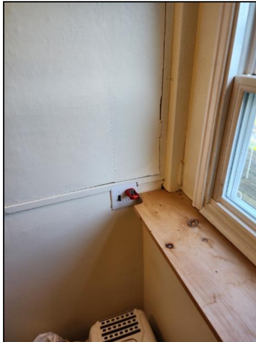
11. Reversed polarity
