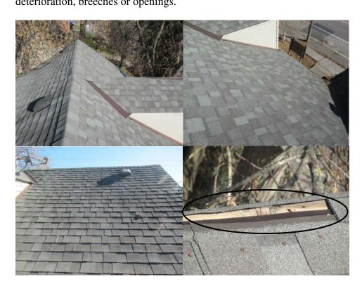
Review. Missing shingle(s) noted at the peak of the front right dormer. Review for repairs, as required, to prevent moisture infiltration into the home.
