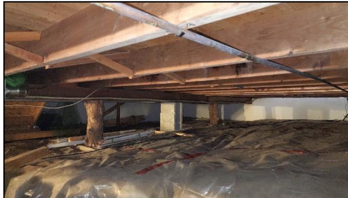
2. Masonry columns
