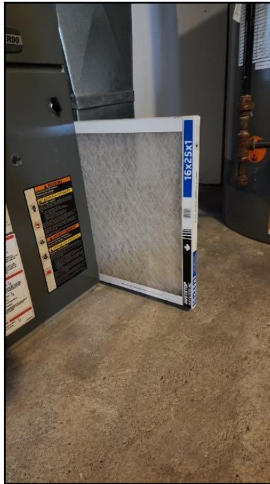
21. Replace - regular maintenance
