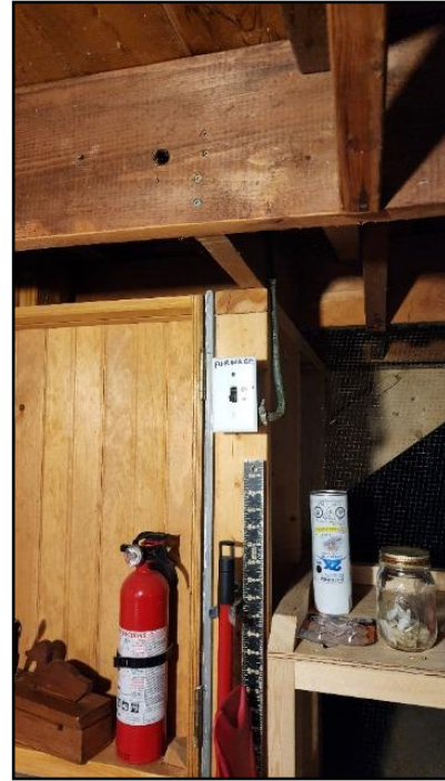
18. Electrical disconnect
