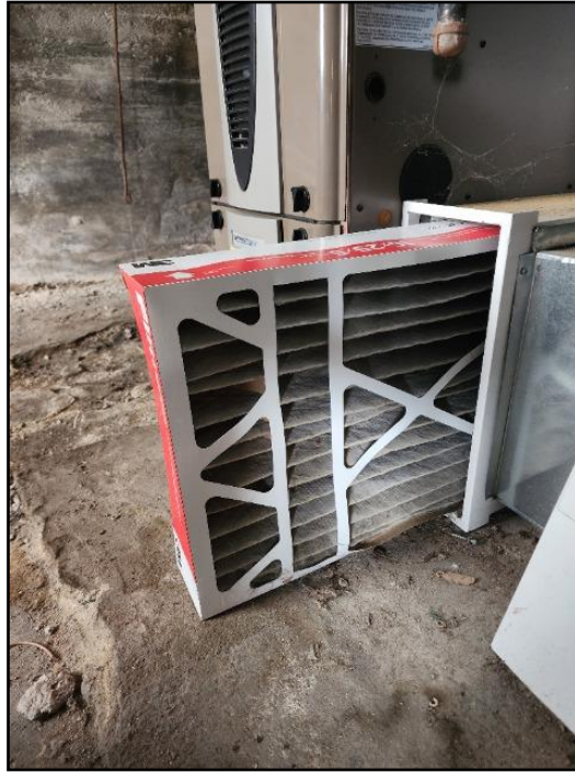
14. Replace - regular maintenance
