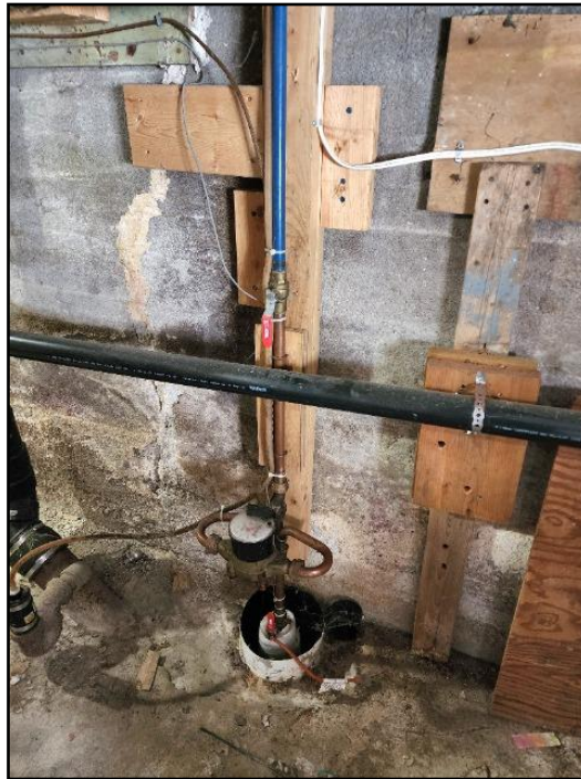
19. Main water shut off
