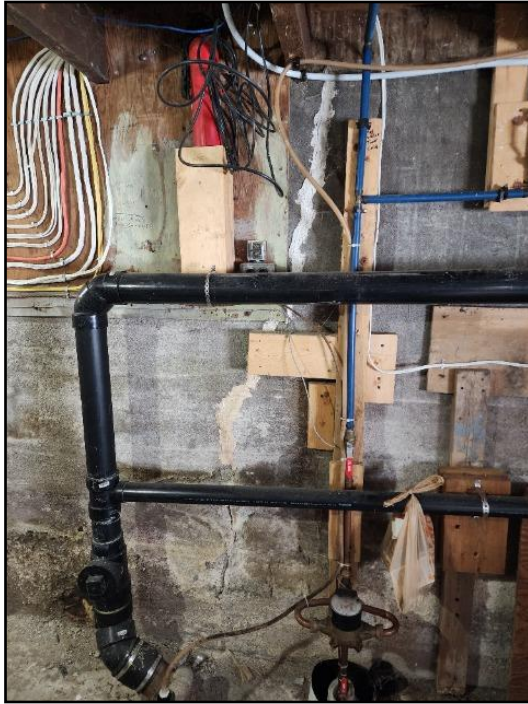
2. Typical minor cracks
