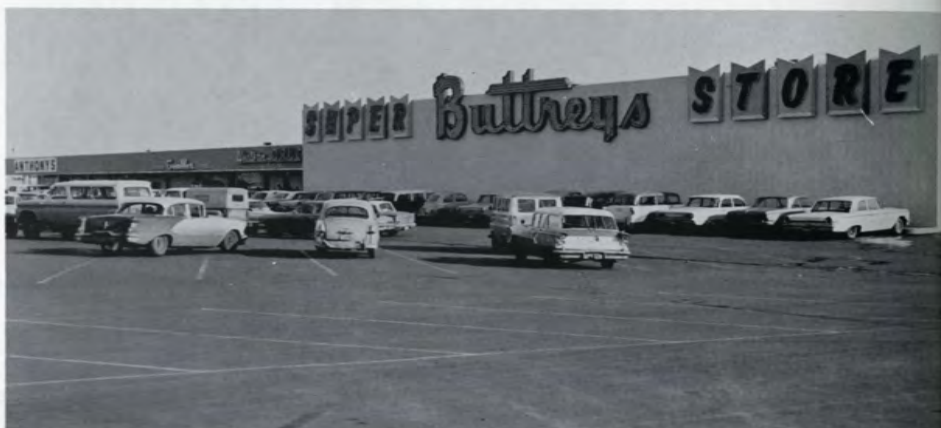
▲ Westgate Shopping Center seen from Northwest.
