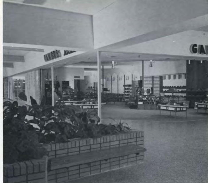
▲ View from the covered mall.
