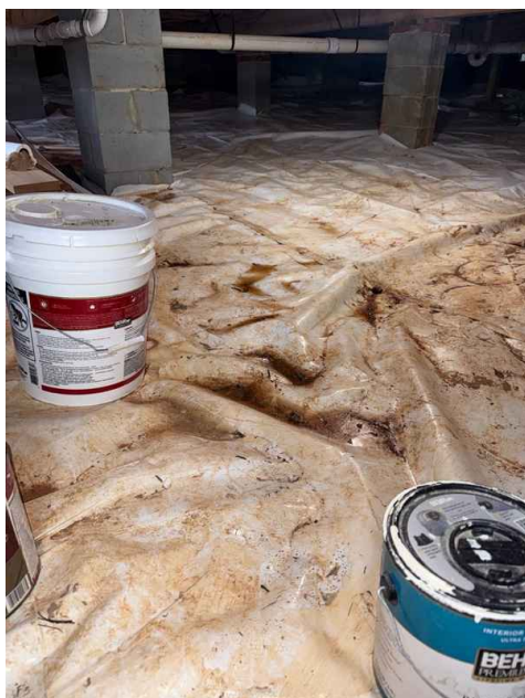
Rear Right Crawlspace
