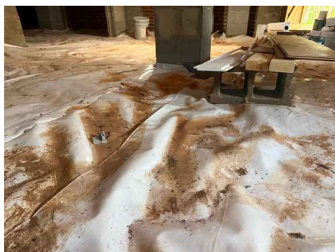
Front Right Crawlspace
