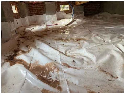
Front Right Crawlspace
