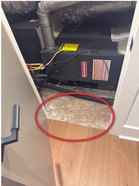
2nd Floor Front Left Bedroom Attic
