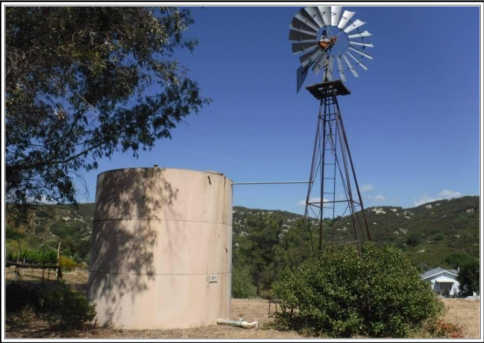
wind pump and tank
