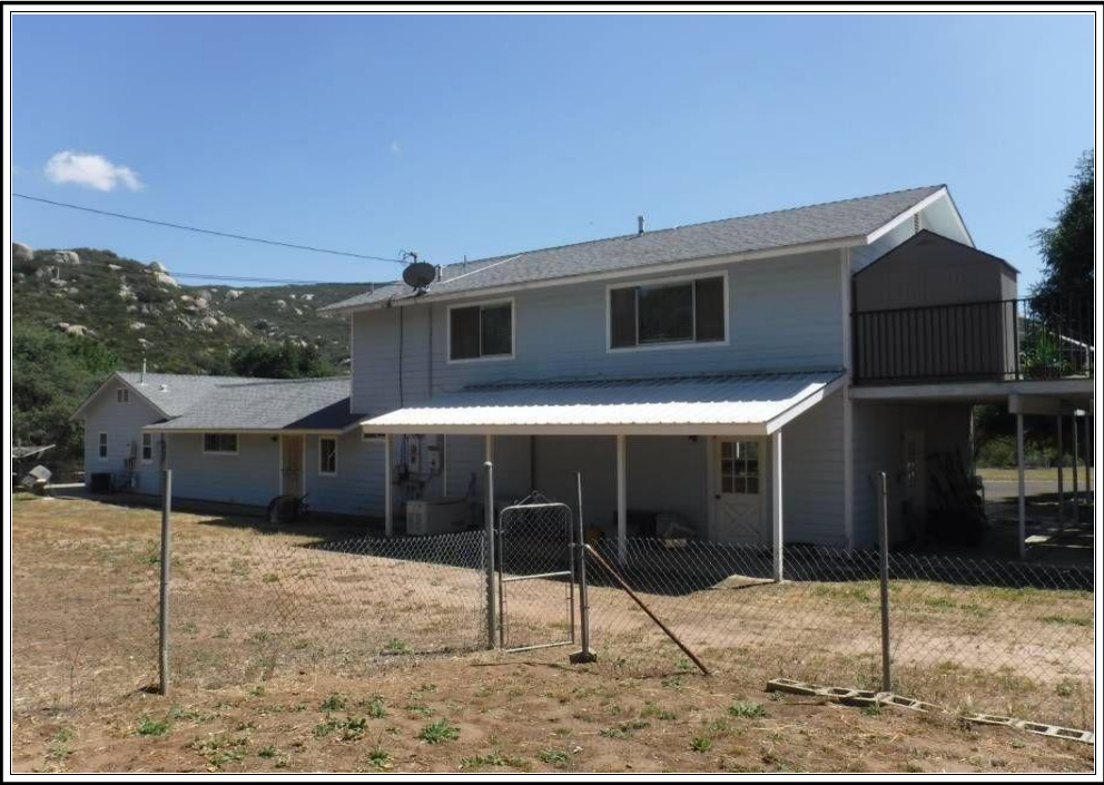
REAR OF SUBJECT PROPERTY
